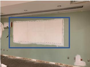
Wall will be mounted to the wall with the rectangle. The patch is  $\frac{34''}{2}$  plywood over 12'' on center heavy duty steel studs.
